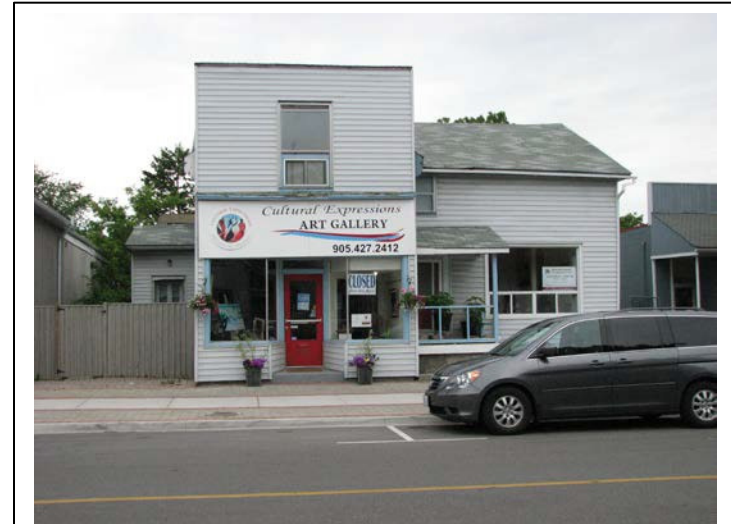
62 Old Kingston Road. A false front on a gabled village building shop mimics the form of a town shop.
