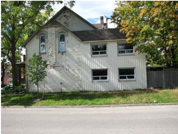
The Linton Avenue frontage of 72 Old Kingston Road provides an opportunity for planting of some street trees.
