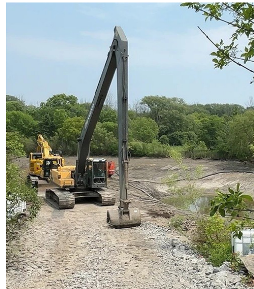
Stormwater Pond Rehabilitation
