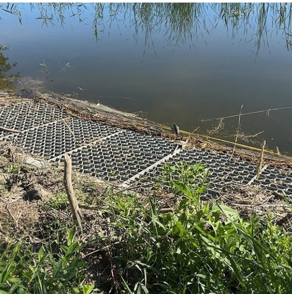
Beaver Dam Removal
