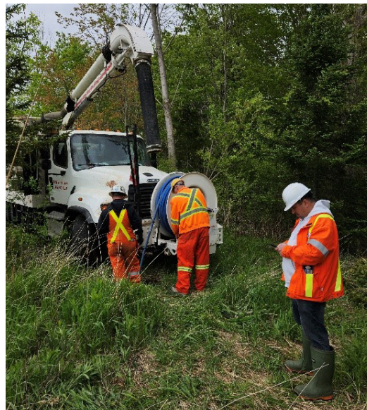
Beaver Dam Removal
