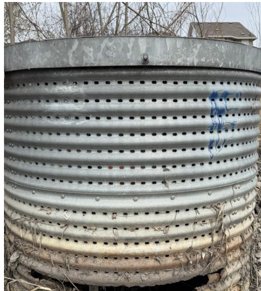
Greenhalf Storm Pond
