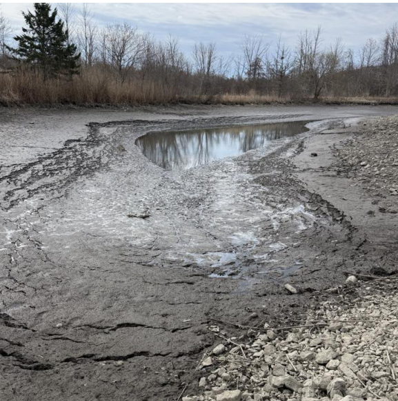
Greenhalf Storm Pond
