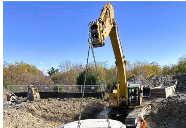
Manhole Installation
