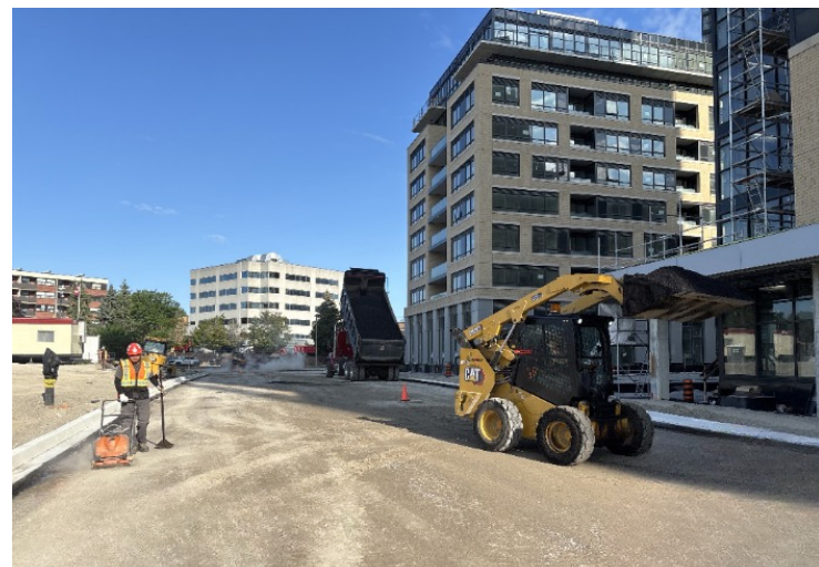
New Road Construction
