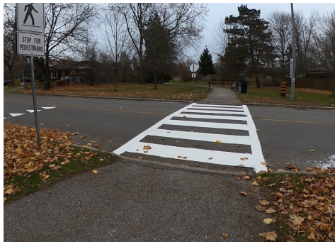
Pedestrian Crossings: New Level 2 Type D Pedestrian Crossover on Clements Road by the Greenbelt Trail (between Burrells Road and Simpson Road)
